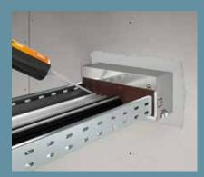
Completely close the cavities with PYROSIT® NG fire protection foam
